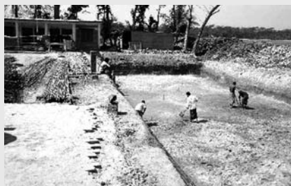
Bangladesh: Grant Aid for Disaster Prevention and Reconstruction
