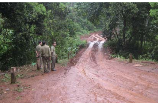
Road close to the national borders of Vietnam and Cambodia, which is difficult for traffic
