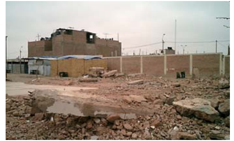
An elementary school immediately after the disaster. The building was thoroughly destroyed.
