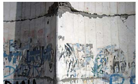
Water tank with visible cracks. As there is danger of the tower collapsing, a new water tower will be constructed in a new site.
