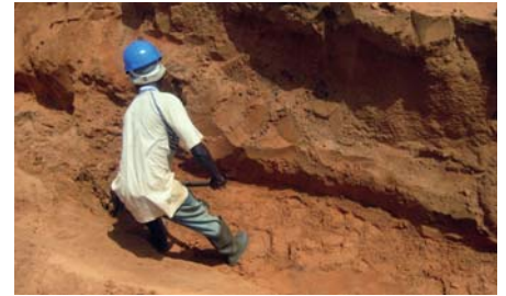
Constructing a school in Senegal
