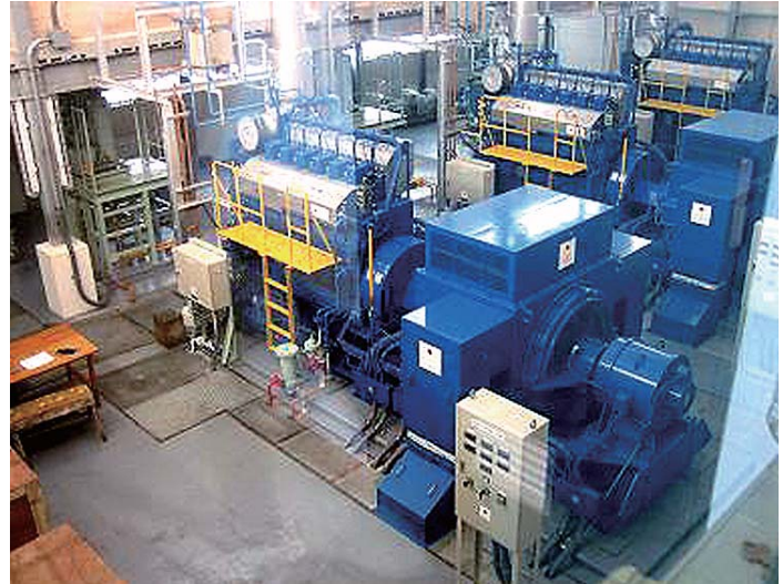
The power station in Tuvalu that uses the diesel fuel provided
