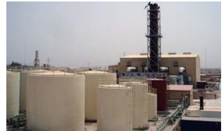
Samawah Diesel Power Station
