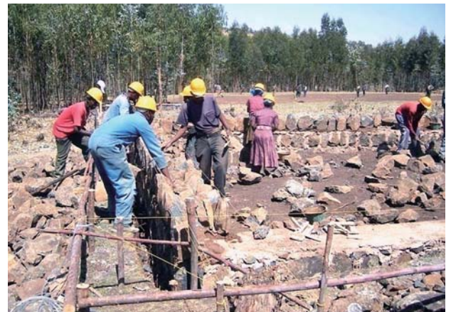
Ethiopia - Foundation works for school construction
