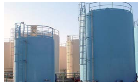
Tank for Samawah Diesel Power Station
