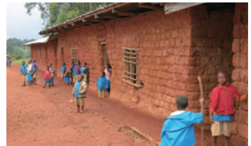
Some of the previous classrooms, built from brick
