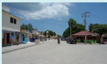
Road repaired following an earthquake (Haiti)
