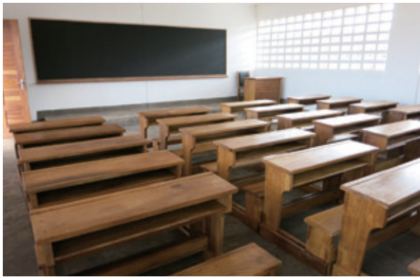
The new classrooms have a brightly lit interior thanks to the use of hollow block windows
