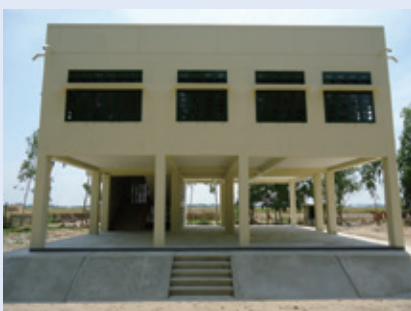
Primary school-cum-cyclone shelter constructed in an area devastated by 2008 Cyclone Nargis (Myanmar)
