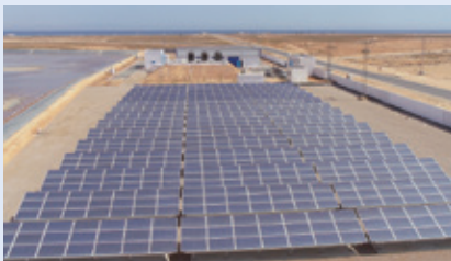
Groundwater desalination plant (white buildings at rear) and solar panels (Tunisia)
