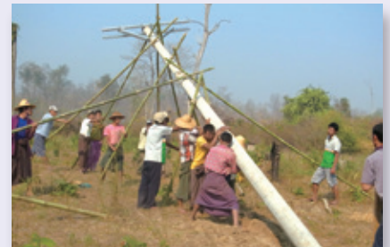
Utility poles were erected thanks to the full-scale cooperation of community residents
