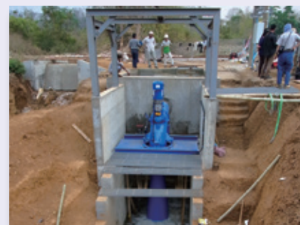
An installed micro-hydro generation unit undergoes test operation
