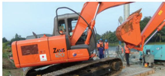
An excavator for river dredging was procured for use in carrying out anti-flood measures (Indonesia)
