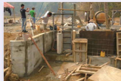
Civil engineering works carried out for a micro-hydro project
