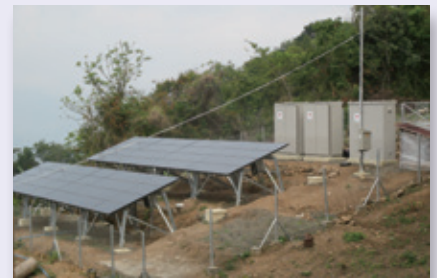
Solar panels and generators
