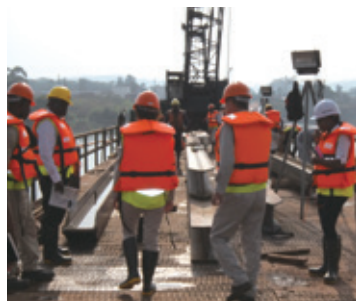
Ex-Post Procurement Audit: Construction site of a project to be audited in Uganda
