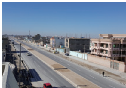
Paved road after completion (Afghanistan)
