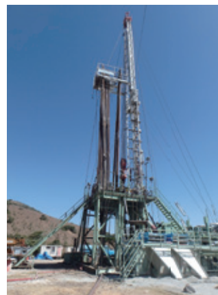
Well-boring equipment (Geothermal power generation project, Ethiopia)
