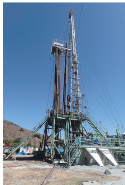
Drilling rig (Forest Preservation Programme)
