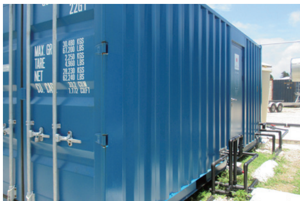
Marshall Islands: Seawater desalination plant for producing drinking water
