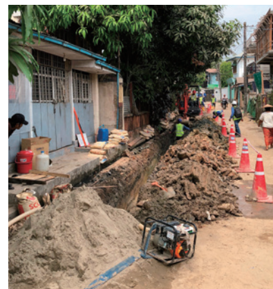
Excavating a road to lay water pipes
