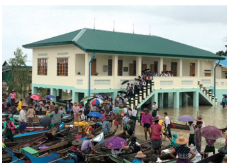
Students leave school by boat from the second floor of a new school building equipped with a flood control structure (Myanmar)
