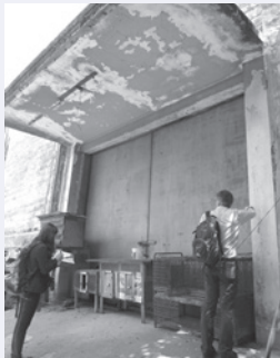
Inspecting an existing warehouse in the Philippines
