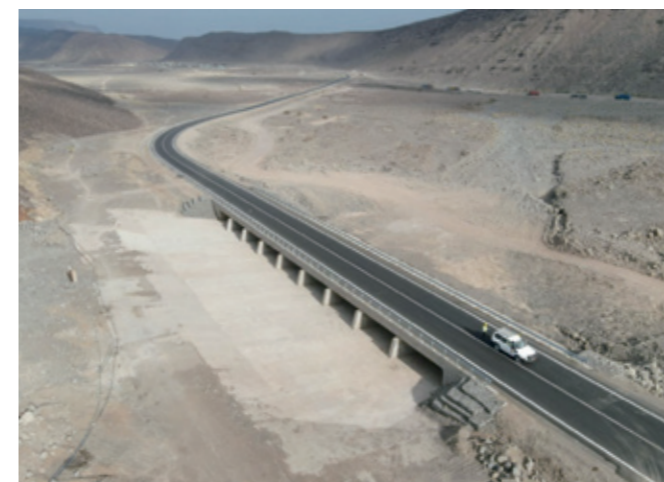
← Nine-span box culverts* (Courtesy of Yachiyo Engineering Co., Ltd.)
