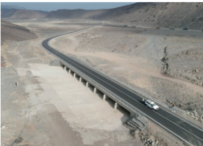
← Nine-span box culverts* (Courtesy of Yachiyo Engineering Co., Ltd.)
