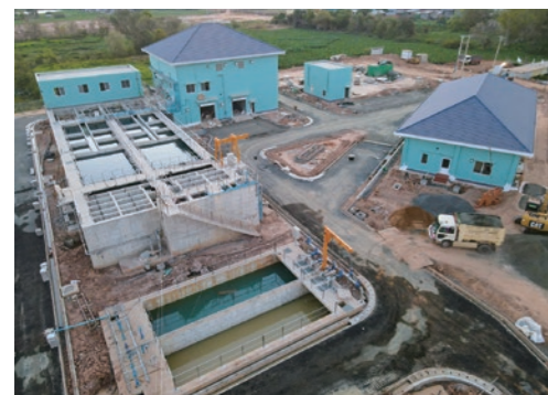
Completed water supply facilities
