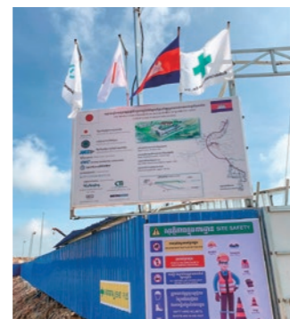
Construction site of water supply facilities
