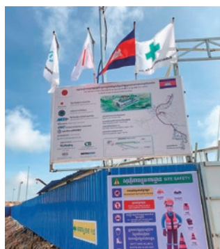
Construction site of water supply facilities
