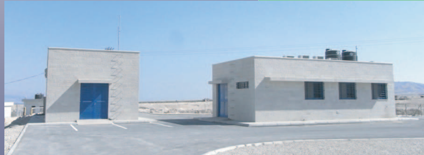
Substation Bldg. & Monitor Bldg.
