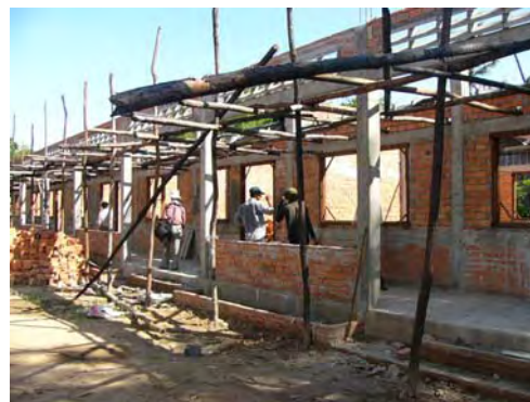
Photo 8: School under Construction
