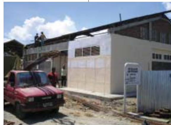
Construction of a fishing lamp workshop in Indonesia
