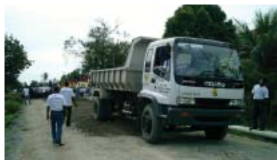
Building an embankment for a road detour
