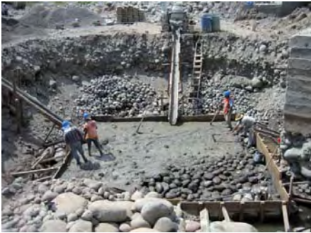
Repair work on a bridge damaged by Hurricane Stan
