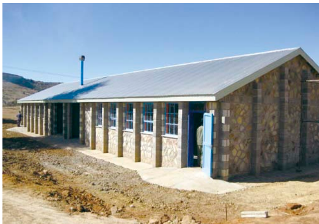
Grant aid for community empowerment: A completed secondary school (Lesotho)
