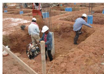
Workers building a roadside station
