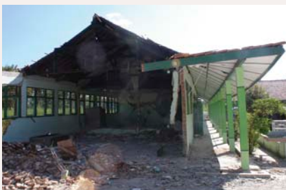
Pungkuran Elementary School immediately after the 2006 earthquake
