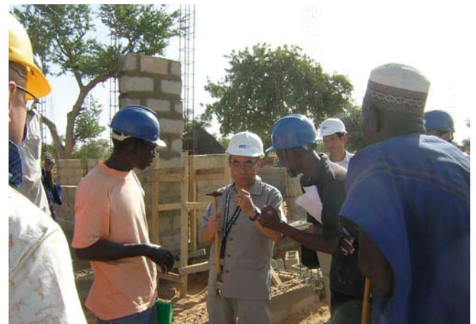
Grant aid for community empowerment: A JICS technical expert carries out construction project management while also providing training to local technical staff (Niger)
