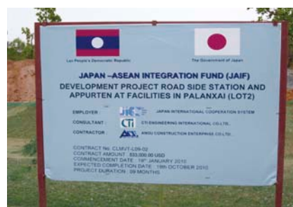
Construction site for a roadside station in Laos
