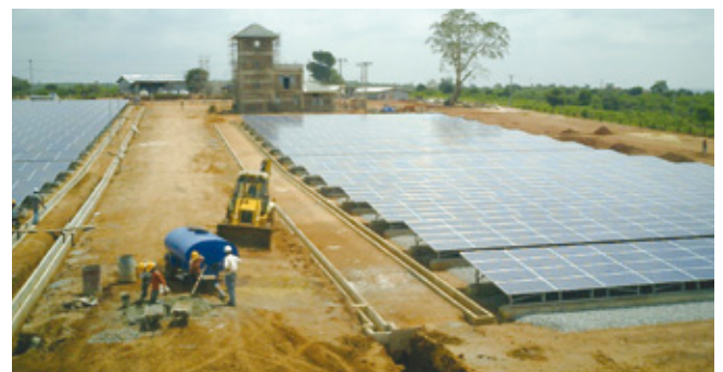
Installation of the solar PV panels and preparation of the site
