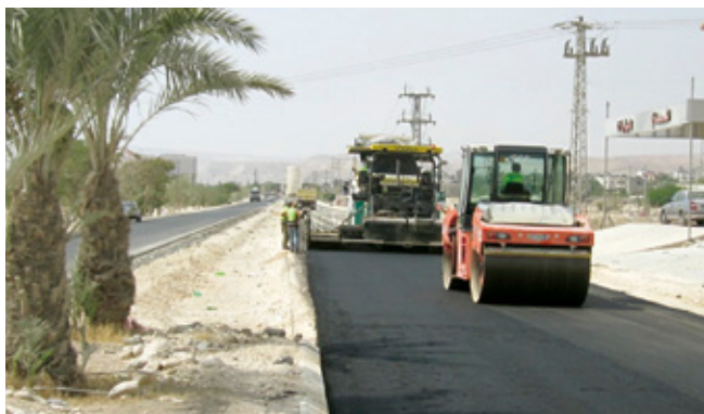
Grant aid for conflict prevention and peacebuilding: Al Quds Street under construction (Palestine)
