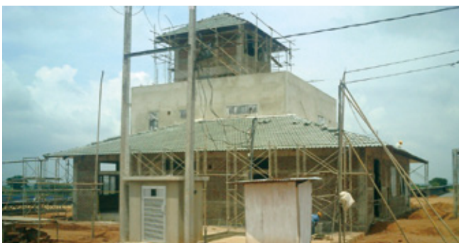
The control building shortly before completion
