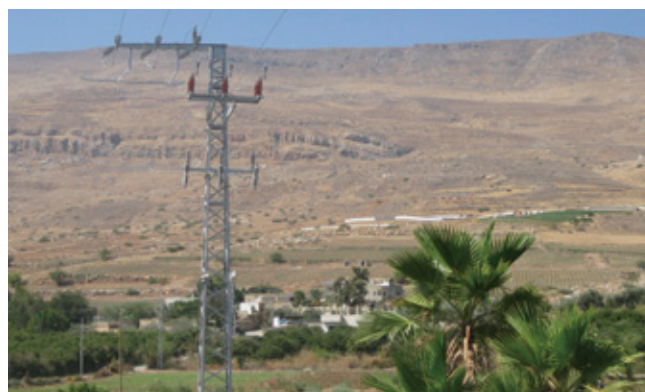
Completed transmission lines and pylon
