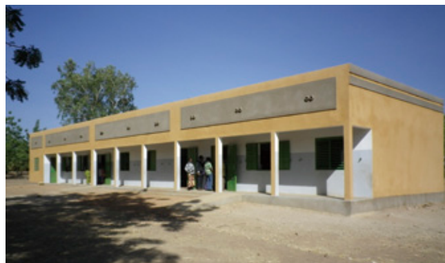
Grant aid for community empowerment: Elementary school that was constructed using grant aid (Burkina Faso)
