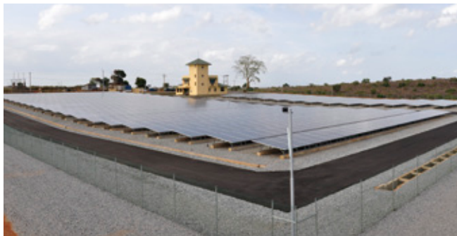
Program grant aid for environment and climate change: Solar panels installed in Hambantota (Sri Lanka)
