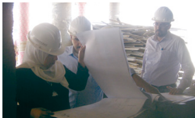
Palestinian consultants check plans while overseeing construction works
