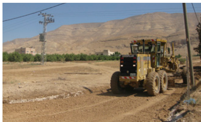
Road repair work being carried out (foreground) and completed electrical transmission lines (background)
