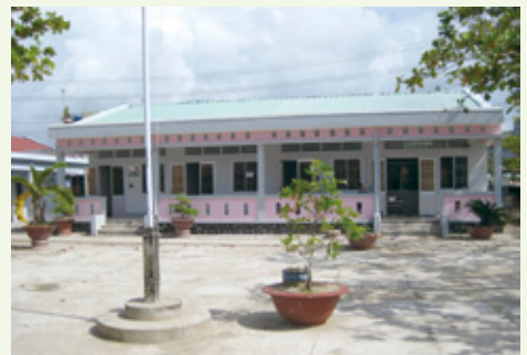
A completed health center (Vietnam)
