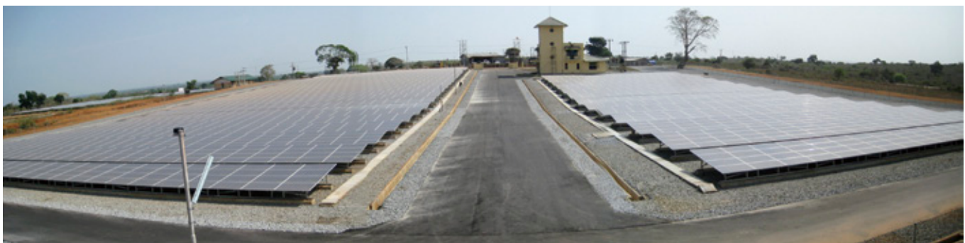
The solar PV panels laid out in neat rows during the installation work
