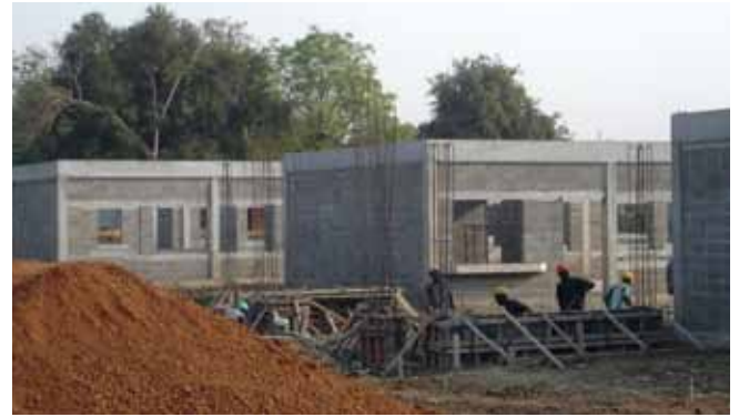
The MTC in Juba shortly prior to completion
