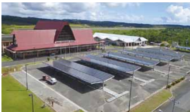
Solar electricity generation system installed at Palau International Airport
