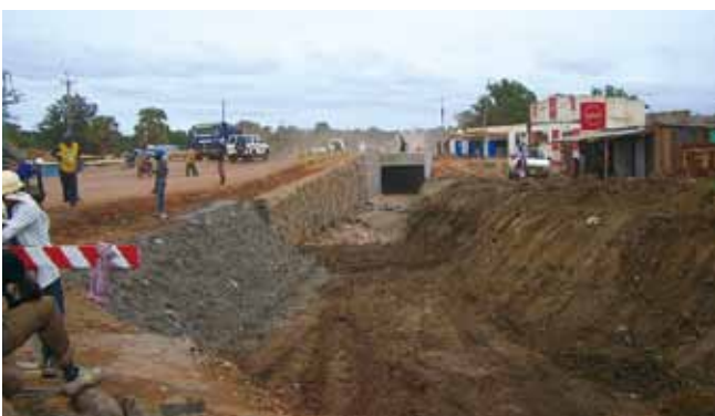
Construction of a channel for culverts in The Project for Construction and Rehabilitation of Bridges on Main Roads in Juba City
