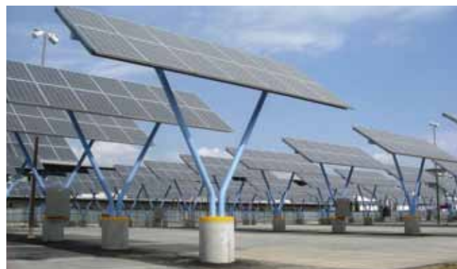
Solar electricity generation system inside Kabul International Airport (Afghanistan)
