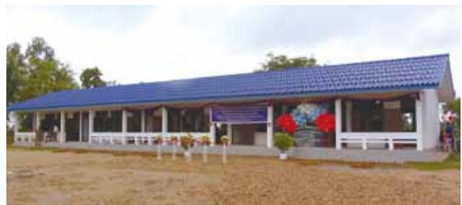
The completed Paksong Lower Secondary School building
