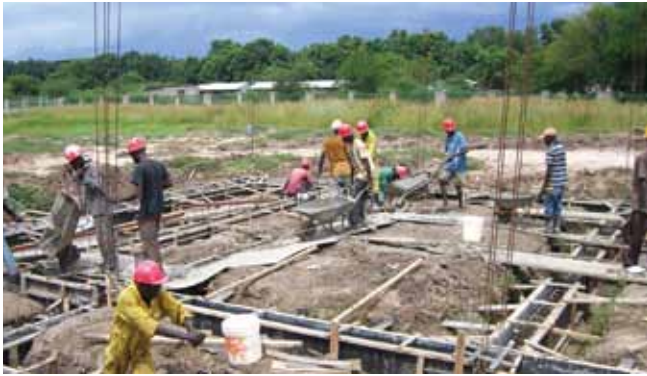
Extension construction work using Grant aid for conflict prevention and peacebuilding begins at the MTC in Juba
