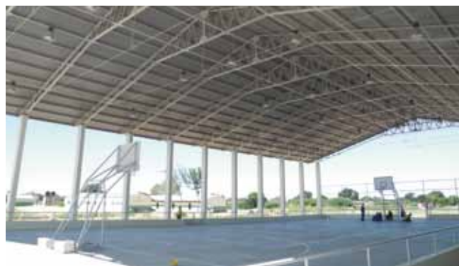
The covered sports facility includes night lighting (Kongolote Secondary School)
