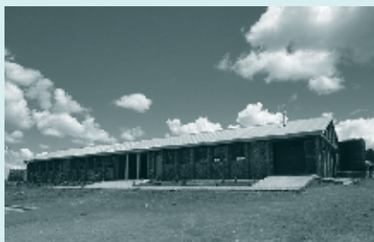
An administration and science laboratory block built with the objective of upgrading secondary school mathematics and science education (Lesotho)
