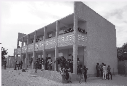
A school building with a slope for wheelchair accessibility (Senegal)
