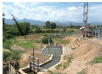
Small hydropower water source site
