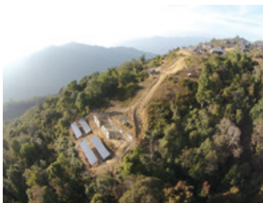
20 kW solar power system
