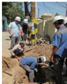
Site pre-inspection in Yangon
