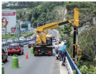
Bridge inspection vehicle used in Guatemala
