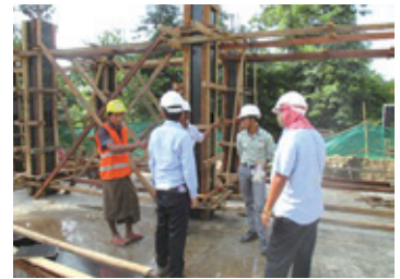
Providing guidance at the reconstruction site
