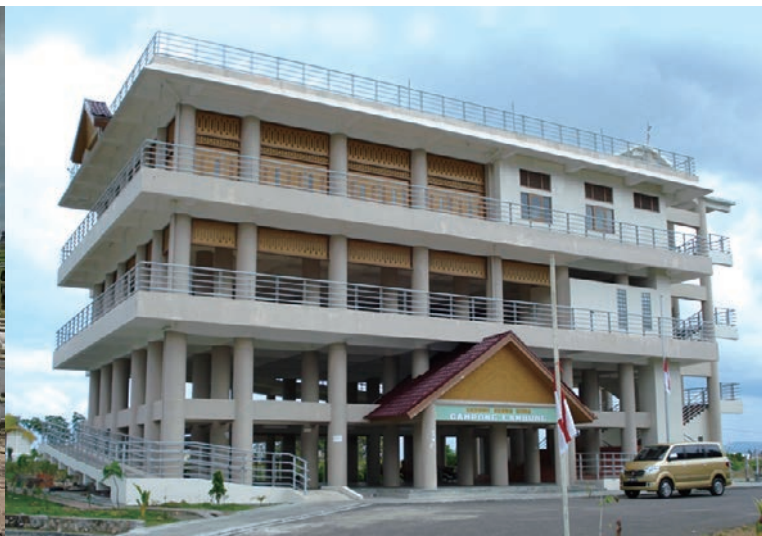
Construction of an evacuation shelter as part of reconstruction assistance following the Indian Ocean earthquake and tsunami (Indonesia, 2009) ↓
