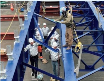
Ukraine — Training on assembling emergency bridges during the Transport Services Phase 2 sub-project
