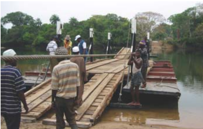
Sierra Leone Boats were repaired, making it possible to transport people and goods again
